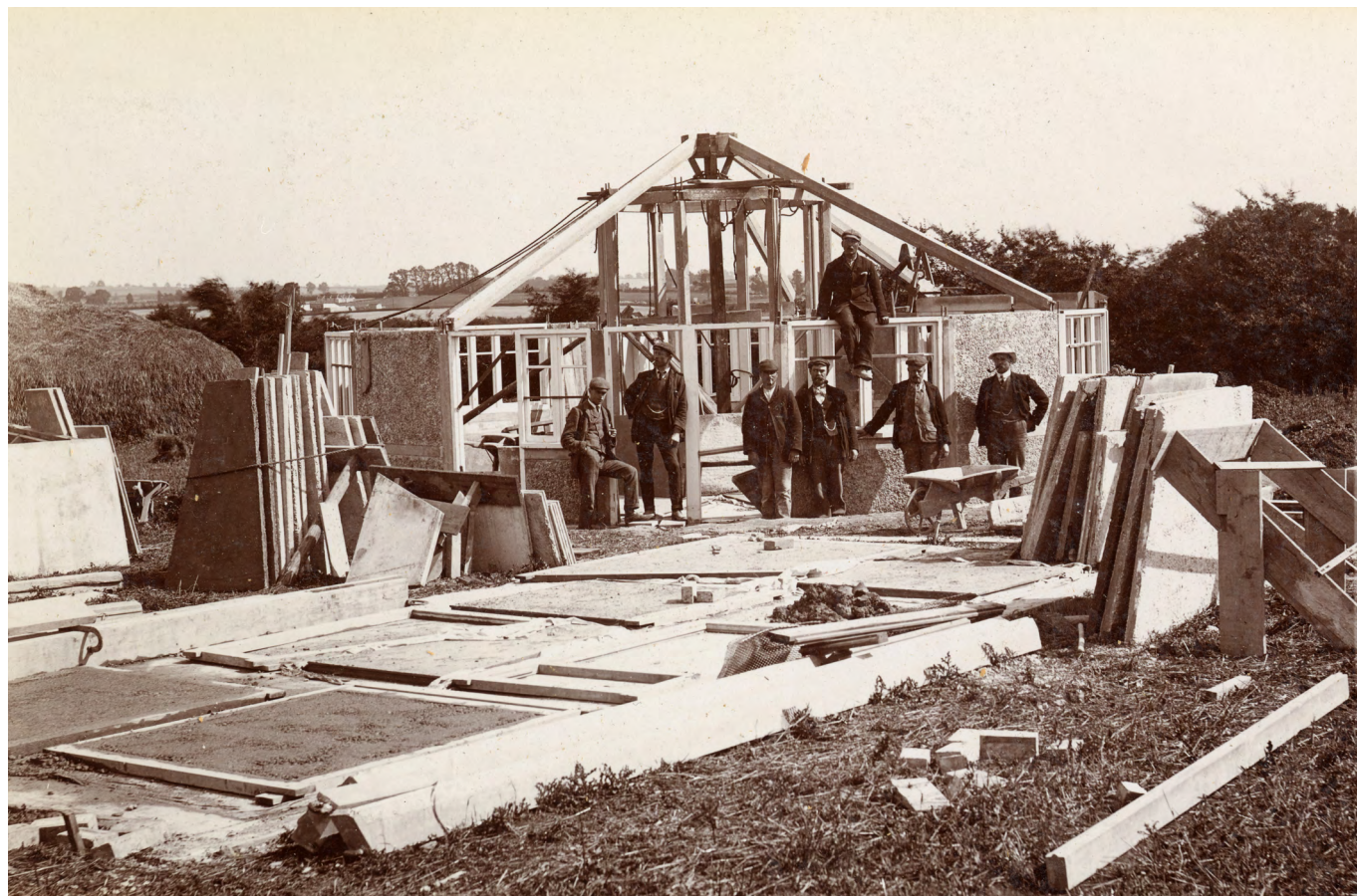
Letchworth Garden Homes. Letchworth, Hertfordshire. © Garden City Collection (Letchworth City Heritage Foundation). Experimental steel framed cottages, as well as avant-garde pre-cast concrete systems and site labour-saving formwork systems using waste materials featured in experimental designs at the 1905 Letchworth Cheap Cottages Exhibition.
