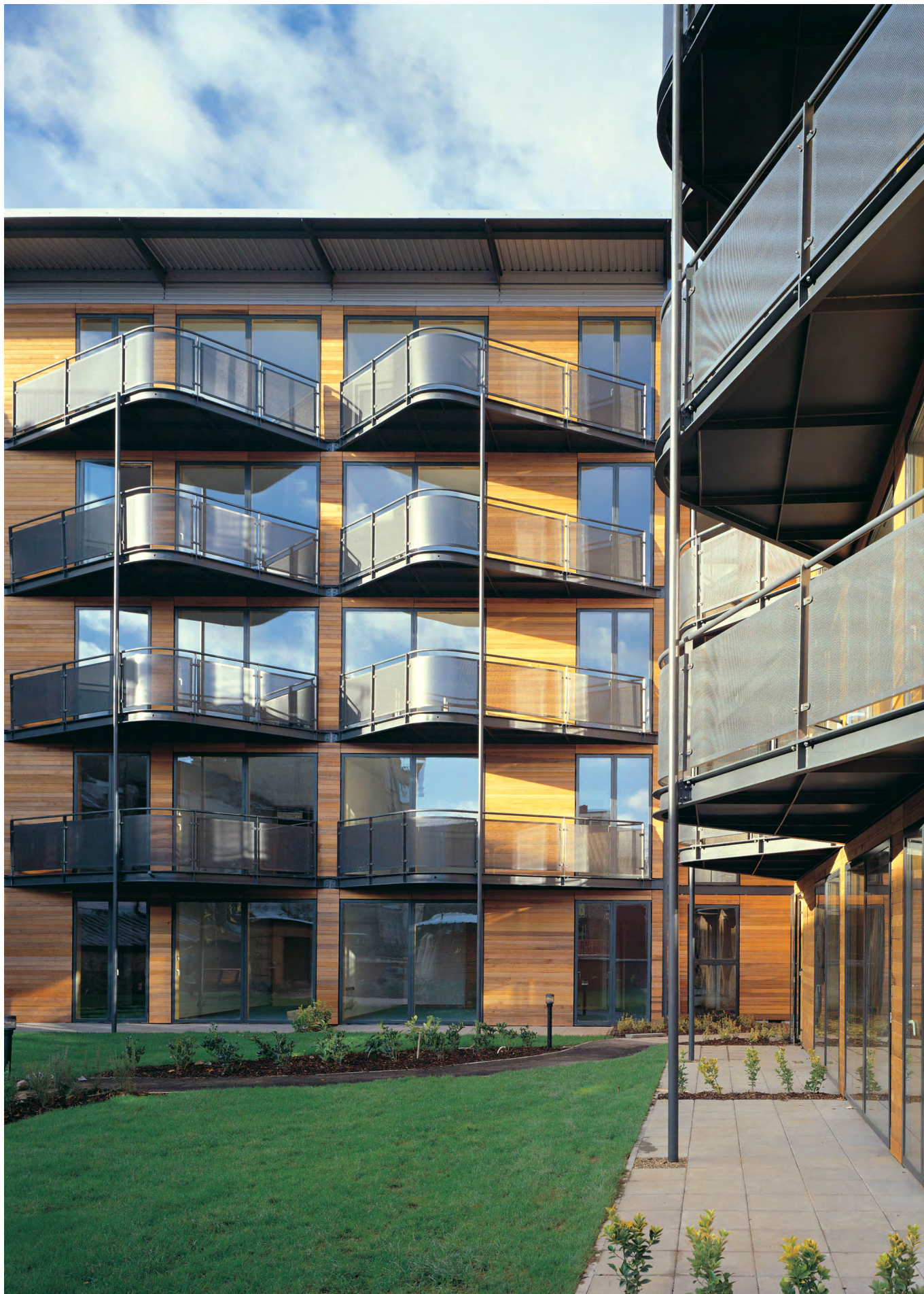
Murray Grove, Cartwright Pickard. Hoxton, London. Photograph: © Martin Charles. An early volumetric scheme for key workers built by Peabody. The timber and terracotta cladding was applied on site but the volumetric units were delivered with all of the bracketry and fixings necessary to receive the cladding. Internally they were fully fitted out and decorated. The attention paid to detailing and the high quality external materials have ensured that this building retains its appeal twenty years after its construction.
